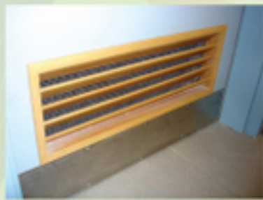
Fig. 6.16 (Left) & Fig.6.17 (Right): Ventilation louver installed with wire mesh.
