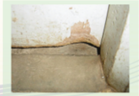
Fig.6.15 Wooden door gnawed by rodents
