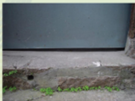
Fig. 6.13 (Left) Threshold clearance of door larger than 6mm allowing rodent passage.
