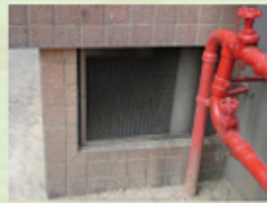
Fig. 6.16 (Left) & Fig.6.17 (Right): Ventilation louver installed with wire mesh.
