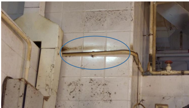
Rat smears on pipe (left) and metal louvre (right).
