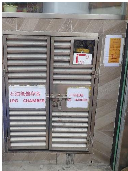
Typical LPG Cylinder Storage Chamber
