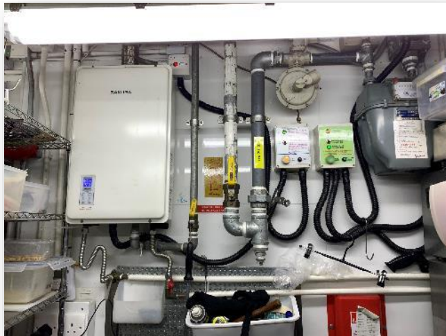
Typical Interlock Device and Indicator lamp
