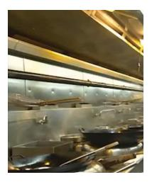
Metal hood properly connected to an air-duct fitted with an extraction fan of adequate capacity shall be provided over all food cooking equipment such as ranges, meat roasting ovens, deep fat fryers and barbecues in the food preparation area. The exhaust shall be arrange to pass through a grease filter, and if required, an air pollution control equipment such as a water scrubber, electrostatic precipitator, etc. before discharging into open air
