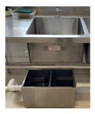
Adequate grease trap shall be provided to separate grease from wastewater so as to prevent the discharge of grease or oil into any drain or sewer
