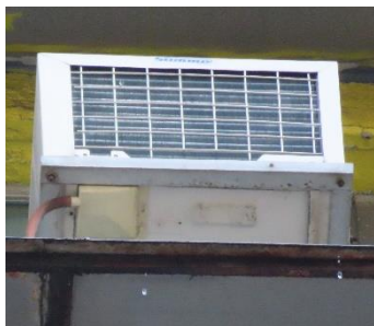
Figures 5 and 6: Wetting of pavements by dripping air-conditioners caused by faulty connection of rubber drain hoses affects environmental hygiene and the cityscape.
