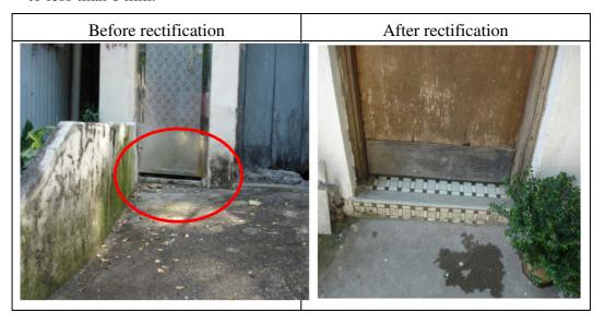
• Fill the cracks in walls, floors and roofs, etc. with sheet iron or cement.
