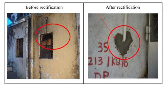
• Install rat guards around the pipes on external walls.
