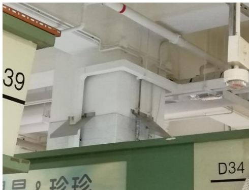
Side branches of piping lets the rodent by-pass the rat guard
