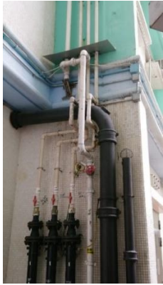
Side branches of piping lets the rodent bypass the rat guard.
