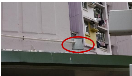
The size of rat guard is too small to screen
