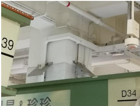
Side branches of piping lets the rodent bypass the rat guard.
